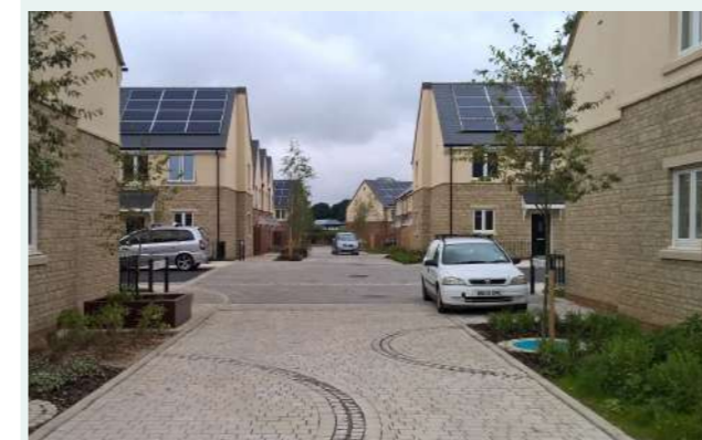
Figure 6.33: Car parking incorporated into the shared surfacing of quieter residential roads.
