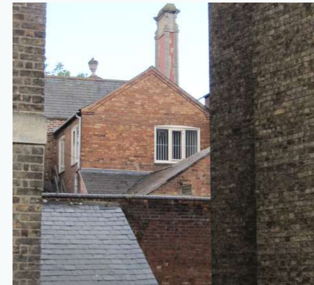
Figure 4.34: The bringing together of a series of simple roof forms creates a rich townscape in Peterborough. Built forms do not need to be complex to be interesting - it is the way that simple forms come together that creates richness
