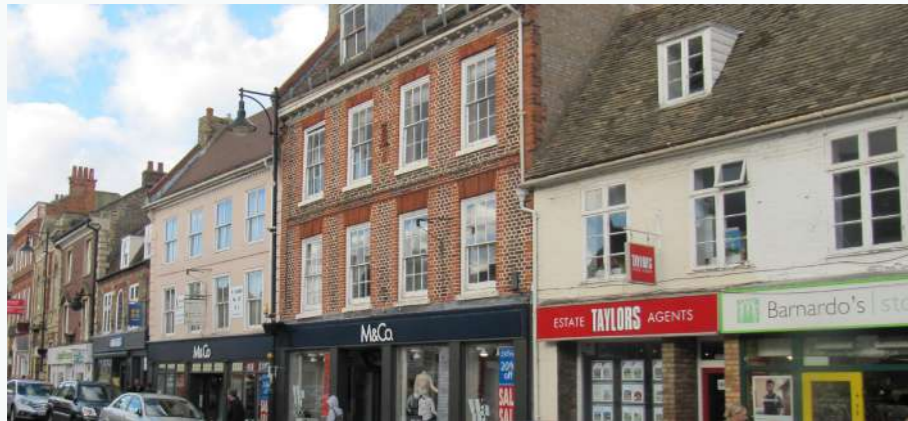
Figure 4.29: Although the building scales and materials vary, the proportions in St Ives Town Centre are similar with a strong vertical rhythm and window proportions consistent across building types.
