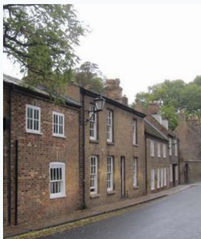
Figure 4.22: Consistent use of a single brick type in Ely brings together these varied building forms.
