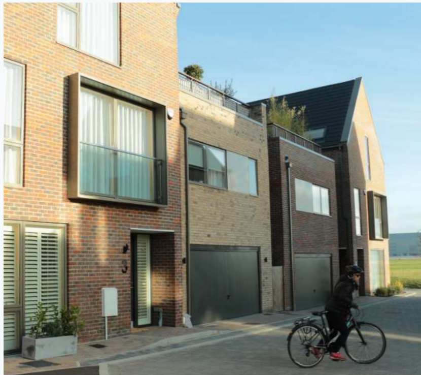
Figure 4.21: Variation in material in this street in Great Kneighton is unified by the symmetrical buildings form, creating a high quality appearance.
