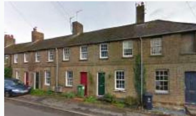
Agricultural brick built cottages in Westwick
