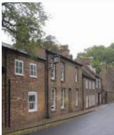
Figure 4.25: Consistent use of a single brick type in Ely brings together these varied building forms.
