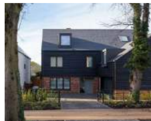
Figure 6.55: On-plot car parking (image above shown space for car parking on driveway and within an integral garage)
